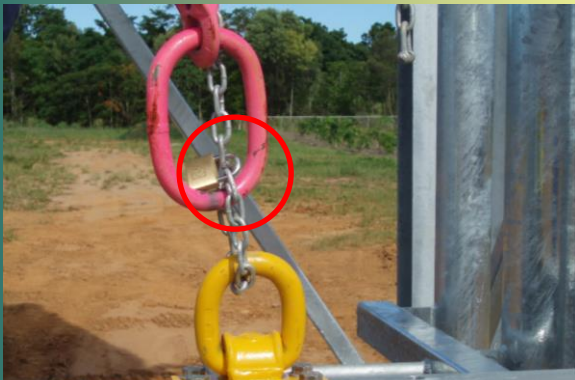
Recovery chain securing master link when tower erected
